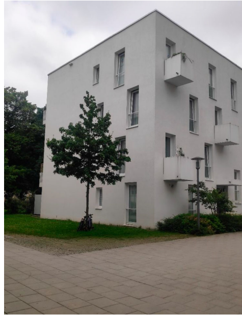
Piusplatz: newly planted tree on underground garage
